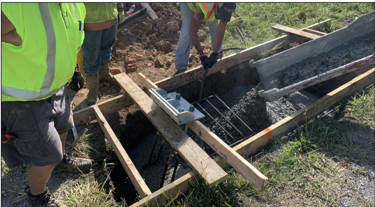
Figure 1: Placement of Anchor Plate
