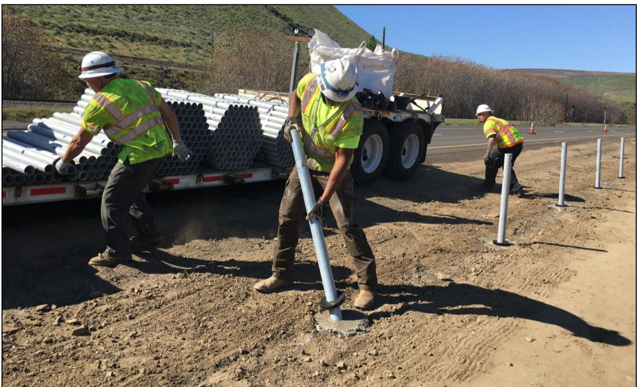
Figure 6: Installation of Line Posts
