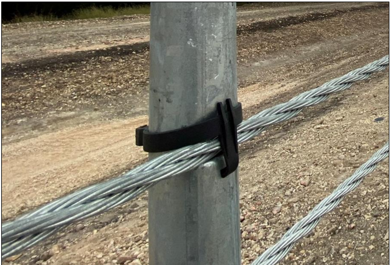
Figure 10: Retainer Clip Position
