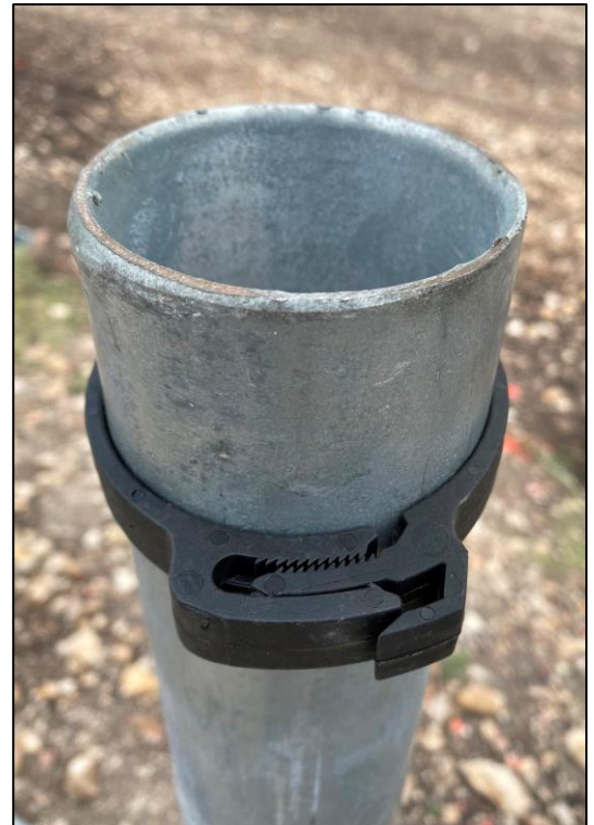
Figure 9: Securing of Retainer Clip
