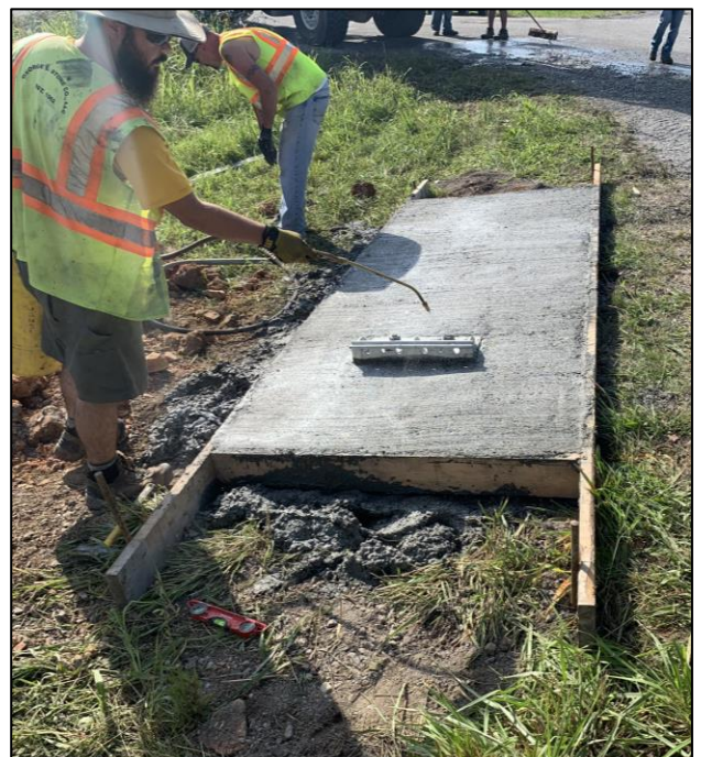
Figure 4: Final Position of Anchor Plate
