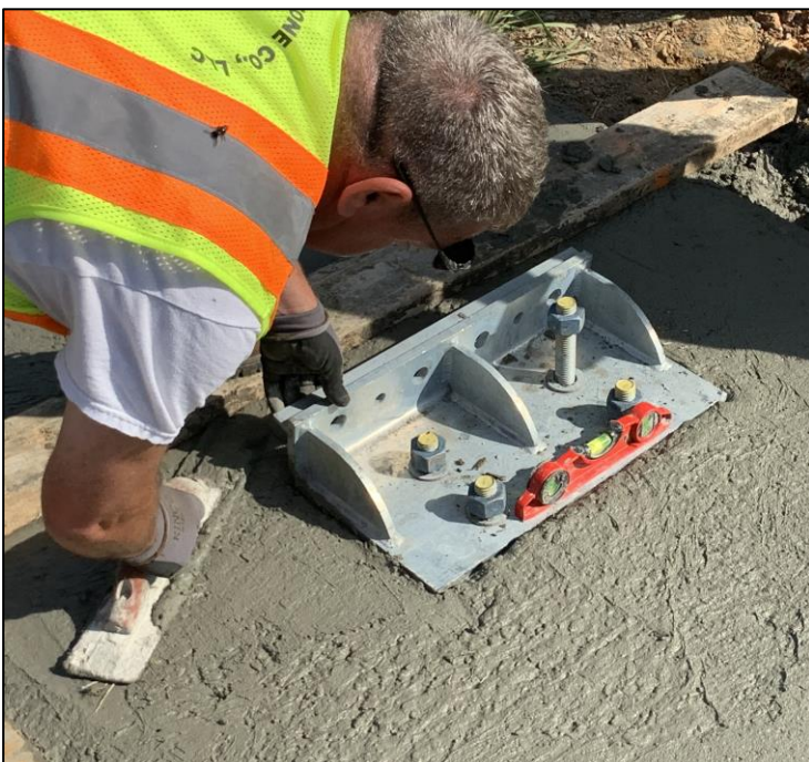
Figure 3: Levelling Anchor Plate
