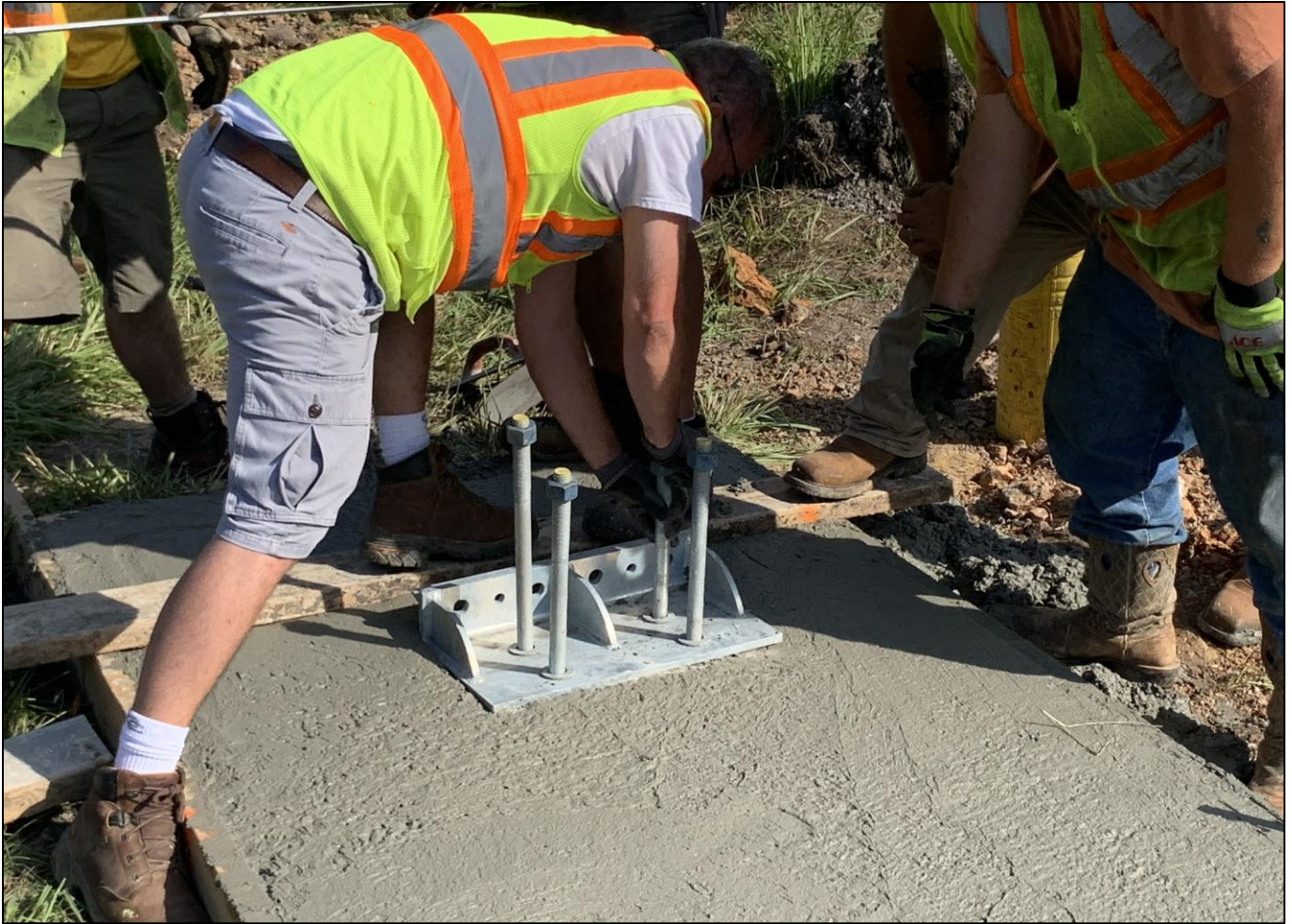
Figure 2: Inserting Anchor Bolts
