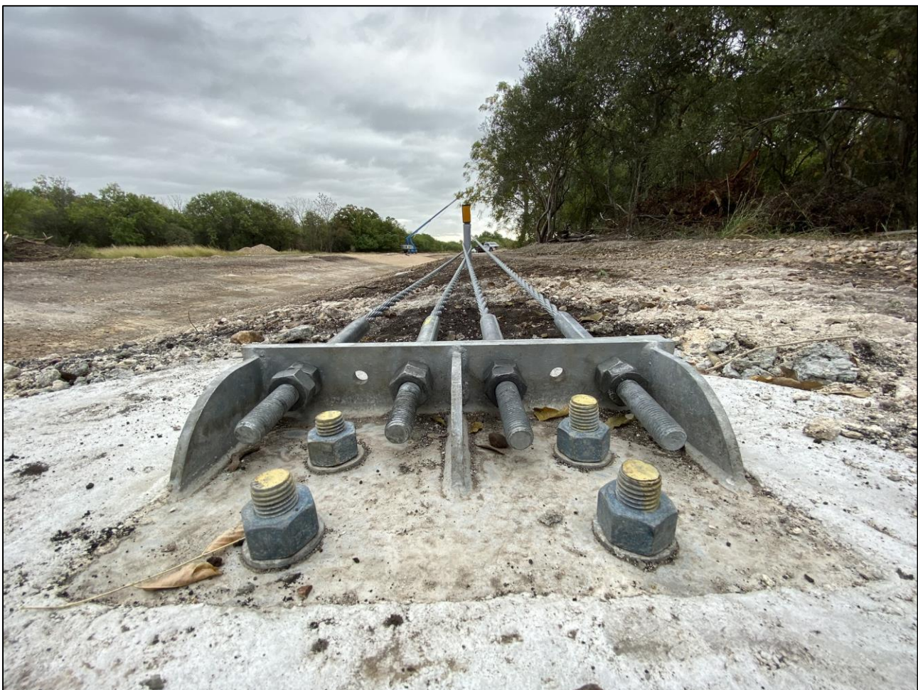
Figure 12: Anchor Bracket Assembly
