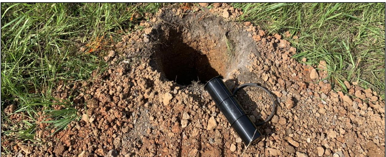
Figure 5: Post Hole with Post Sleeve and Reo Ring
