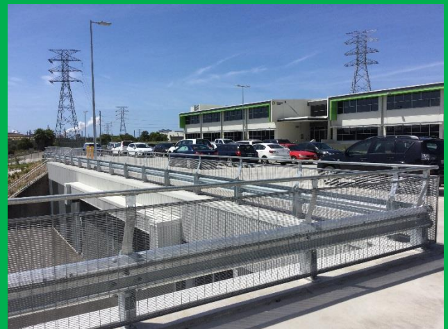
Endeavour Energy Field Service Centre
