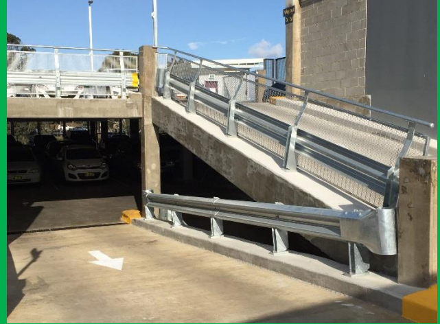
Canley Vale Commuter Car Park
