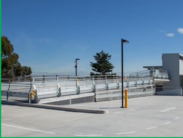
Padstow Commuter Car Park
