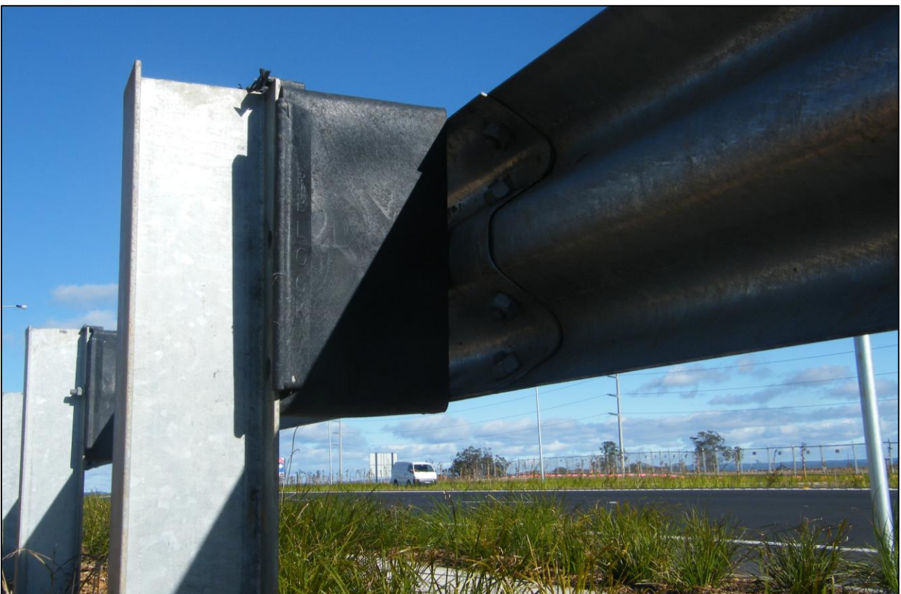
Steel Line Post with 200mm Blocking Piece at Post Location 3
